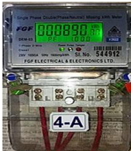
Fig (4) Single-phase smart meter.
