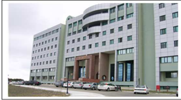
FIGURE 1. A general view of Balikesir University Rectorate Building.
