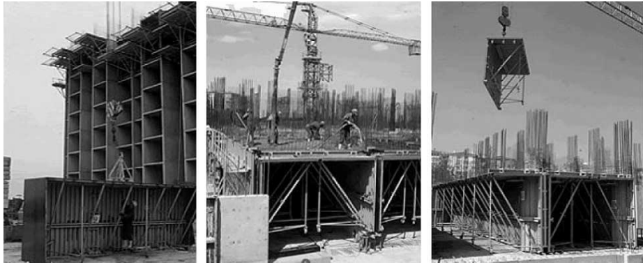
Fig. 1. Tunnel form construction and formwork system.
