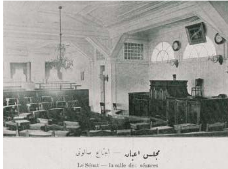
Meclis-i Âyan Hall, Cemile Sultan Palace
