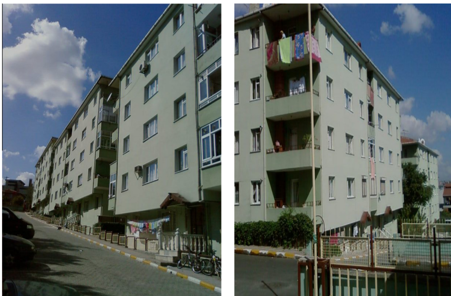
Fig. 1. Observed RC buildings.
