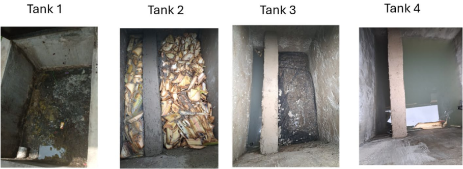
Fig. 8 Developed prototype filtration system in operation and maintenance. The main maintenance activity involves monitoring the filtration performance of the banana stem layer, which is replaced when its color turns dark. Based on initial iteration evaluation, a 9-month replacement interval was established. (Source: Authors Documentation)
