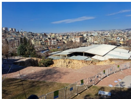
(a) Gaziantep/Sahinbey landslide
