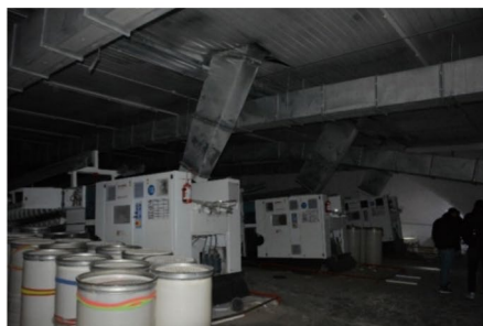
Fig. 28 Damages to non-structural elements (siding damage and machine-equipment damage) in a textile facility in Kahramanmaraş
