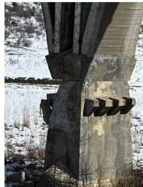
b) Railway bridge - artwork and pier damage
