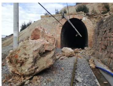
(c) Closing of the tunnel entrance and damage to the tunnel structure due to rockfall and landslide at the railway line tunnel entrance
