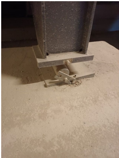
(c) Damage to the pipe support
