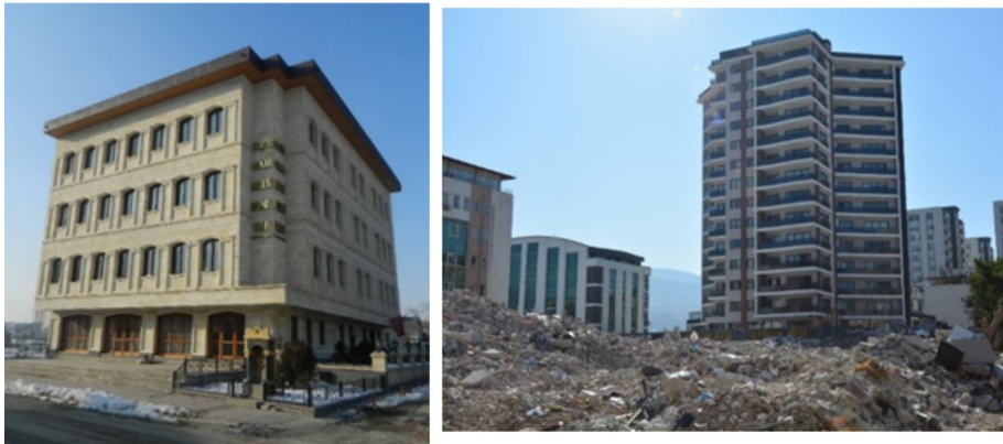
Fig. 26 Undamaged structures after the earthquake
