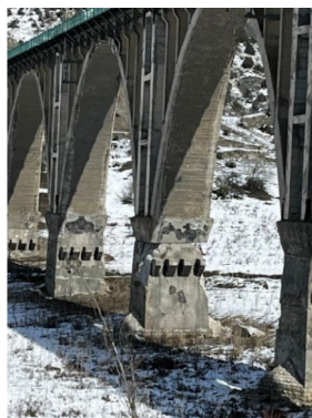
b) Railway bridge - artwork and pier damage
