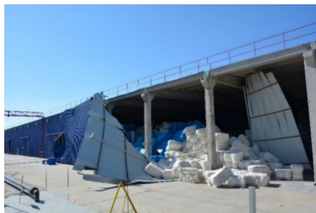
Fig. 28 Damages to non-structural elements (siding damage and machine-equipment damage) in a textile facility in Kahramanmaraş
