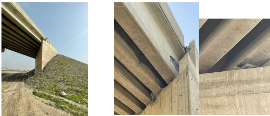
(b) Nurdagi railway bridge: beam damages at the side abutment
