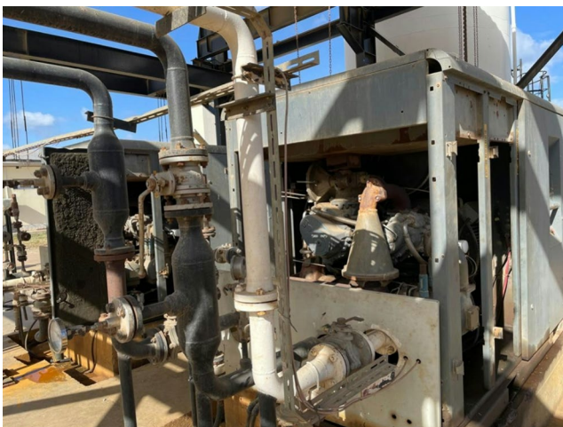
Fig. 2 The real photo Atlas Copco ZT75 screw compressor unit
