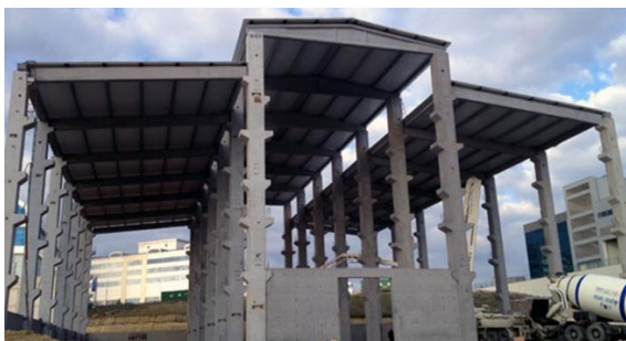
Figure 1. Corbels in an industrial building.
