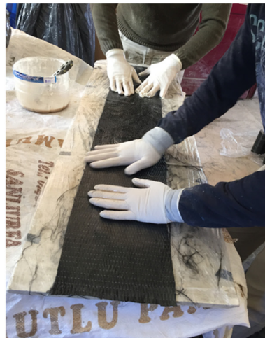
b) FRP sheets preparation
