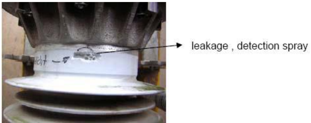
Figure 5. Leak detection utilizing detecting spray.
