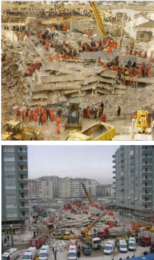
Fig. 1. Progressive collapse of Zumrut Building.
