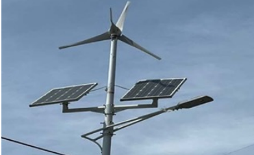
Visual 7. Solar Street Lighting with Solar Energy and Wind Turbine
