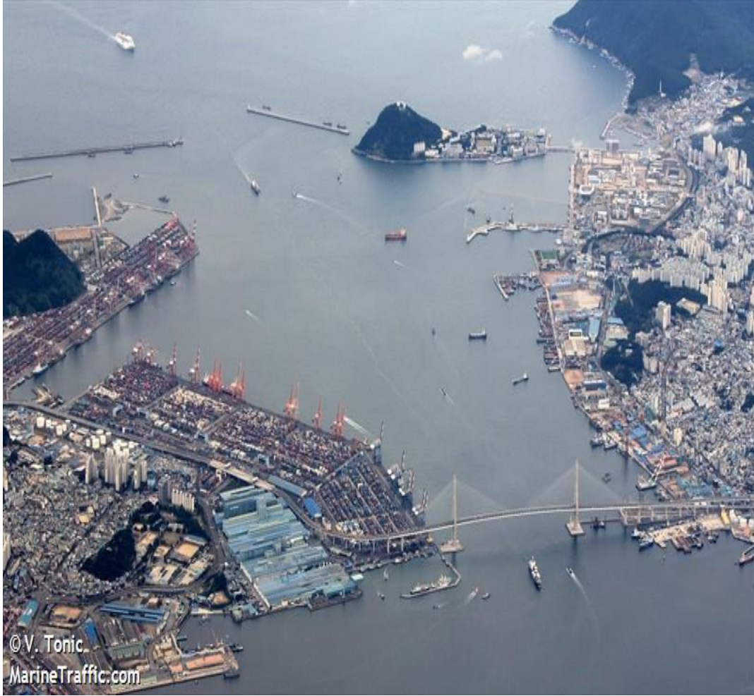
Resim- 9: Busan New Port Distripark 107
