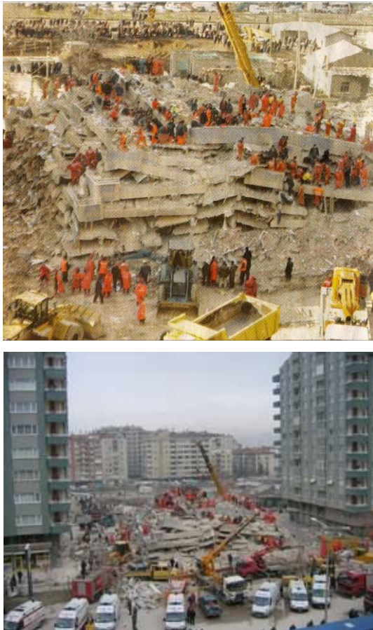
Fig. 1. Progressive collapse of Zumrut Building.
