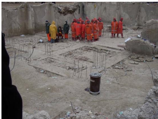
Fig. 7. Continuous foundation system in both directions.
