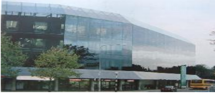
Resim- 4 Briarcliff House, ARUP, İngiltere, (Akıllı Kabuk, Çift Kabuklu Cephe Uygulaması), (Briarcliff House, ARUP, Great Britain) (Smart Shell, Application of Double Shelled Wall) 16
