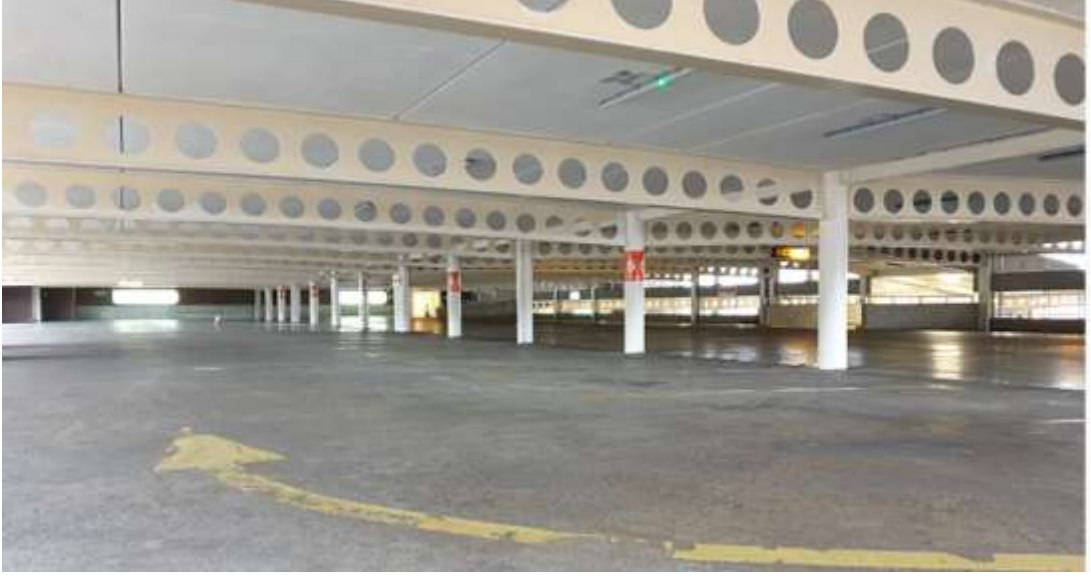
Şekil 13. Otopark Garajı ( https://www.triflex.co.uk/buttercrane-shopping-centre-newry )
