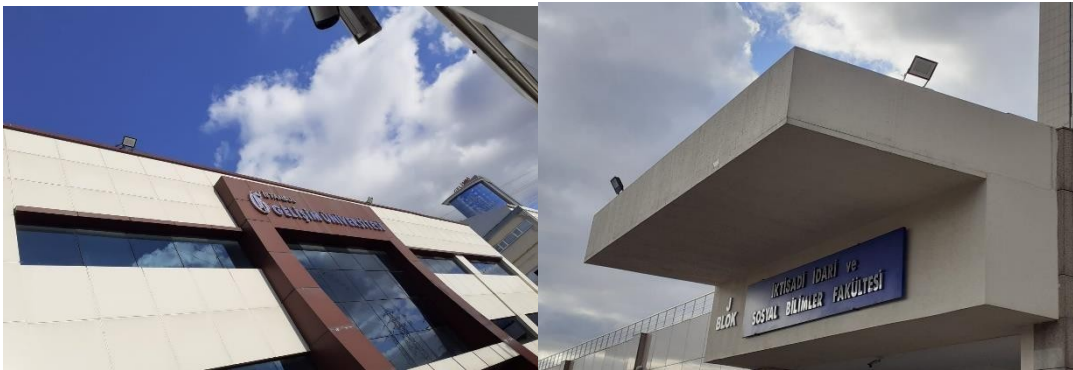
Picture 3. Some areas where we use LED projectors in environmental lighting
